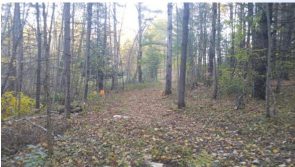
Widening of trail C7B took place in the woods north of Pannis Rd, Town of Wright.
