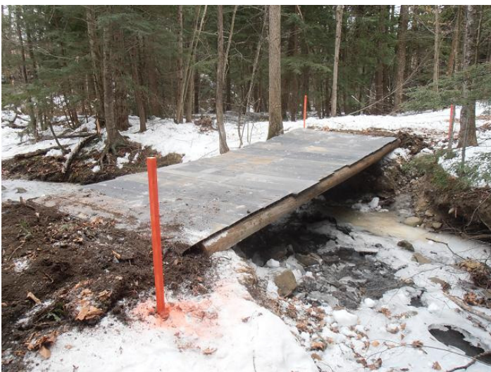
The old bridge on S73 has been replaced by culvert tubes.
