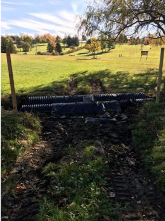
The bridge in Knox Town Park has been replaced
