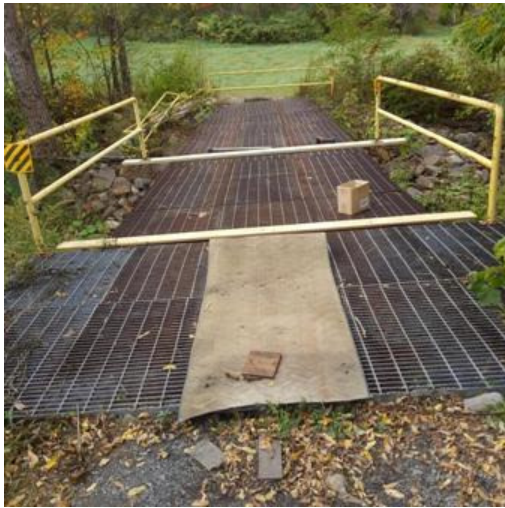
The S72 steel deck bridge now widened, is awaiting pressure treated wood decking.
