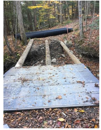
The old bridge on S73, trail to Maple Inn on the Lake, is being removed in this photo.
