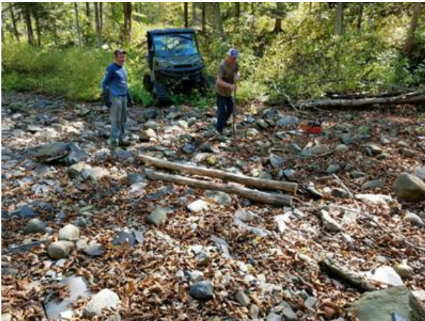
Sept 27th, Joel Church and Laudy Hoyenga work the south bank of Irish Creek. (photo by Tom Rulison)
