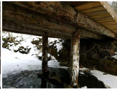
New bridge supports put in place on the Cole Rd bridge in Delanson. Photo by Tom Rulison
