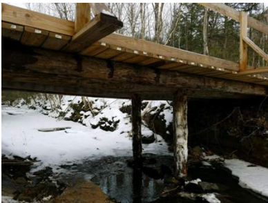
New bridge supports put in place on the Cole Rd bridge in Delanson. Photo by Tom Rulison
