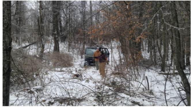
Cutting open a very old logging road on the C7E reroute.
