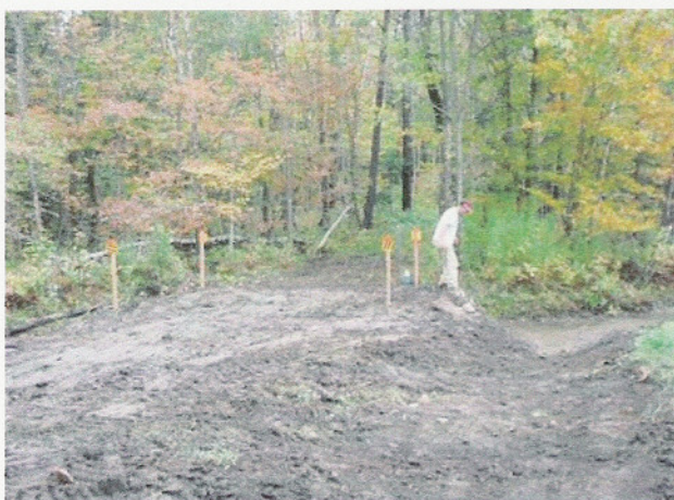
Culvert installation completed in Berne.
