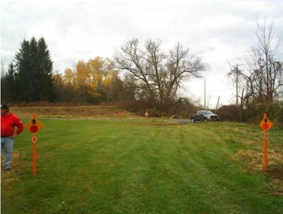
Matt Harper installs a Stop Ahead sign near lower Shellstone Rd.
