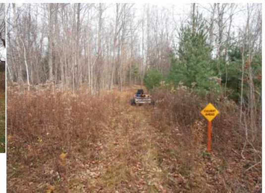
Brushing, clearing and signing on C7B above Gallupville.
