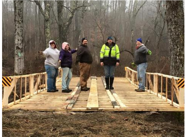
Bridge complete! Brian Buchardt and crew got it done. 40' long, located near Joslyn School Rd.
