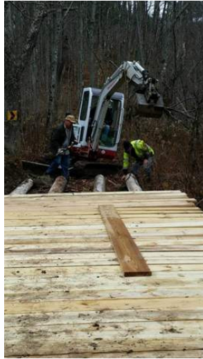
New decking goes on the bridge.
