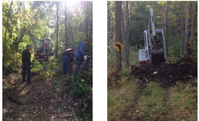
Culvert work on S72 near the Old Maple Inn. Photos by Trail boss Brian Buchardt.
