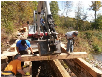
Scott Riley, Tom Rulison and Ray Plant drill set holes in the wood beams..
