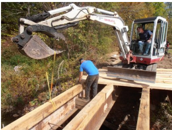
Karl Pritchard positions the beam on the steel girder, then grabs some decking boards with his excavator.
