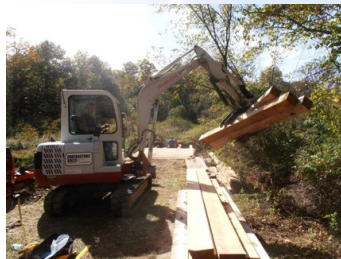
Karl Pritchard positions the beam on the steel girder, then grabs some decking boards with his excavator.
