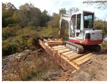
A major bridge over the Normanskill on C7B in Dunesburg was re-decked September 26.
