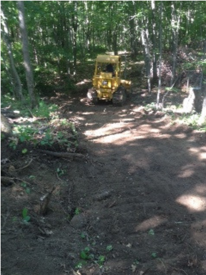
S-72 trail heading to Thacher Park is widened here by Karl and his dozer.
