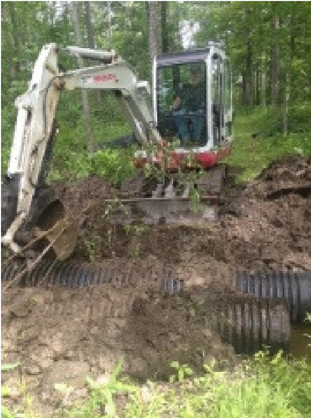
Over on Sawmill Rd Karl, Pat and Brian installed a couple of culvert tubes to S72.
