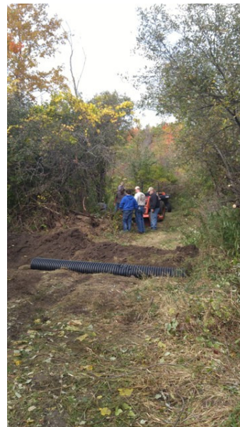
A culvert ready for back fill.
