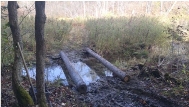
Telephone pole frame will handle the light duty bridge.
