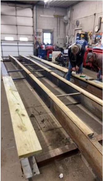
Applying deck nailers.
