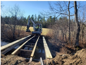
Moving the frame into place.
