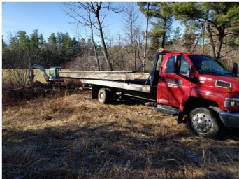
Transporting the frame.
