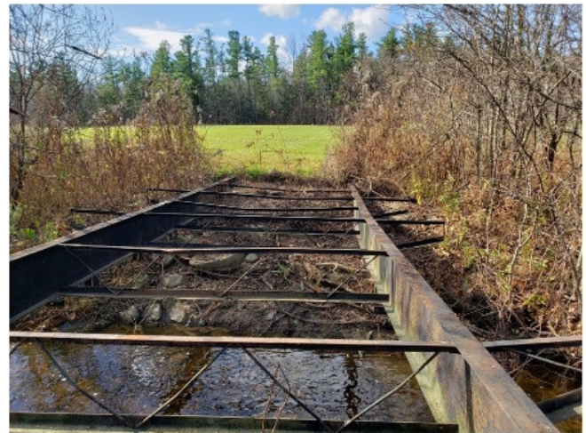
Old trailer frame bridge ready for replacement.
