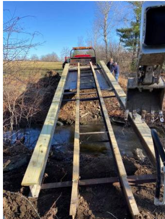
Unloading the I-beam frame.
