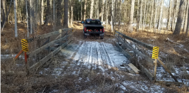
Rt 146 bridge on trail C7B had decking and railings repaired.
