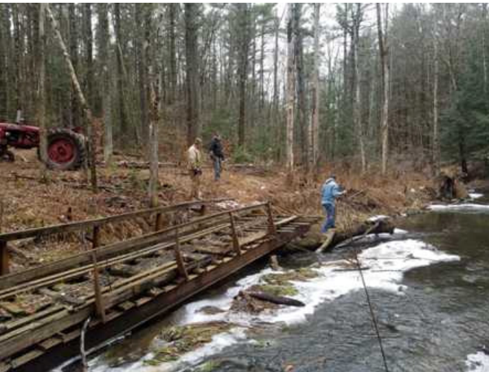
Working with a 40' bridge in the woods is not easy.
