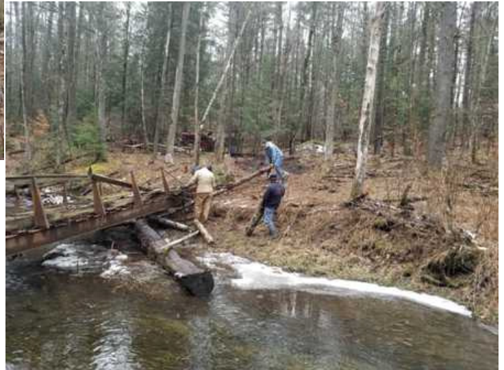
Hoisting the bridge up into position.
