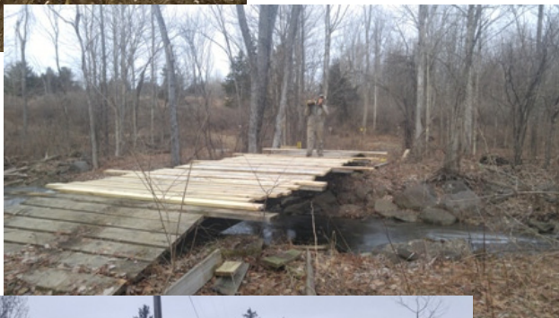
Below: Matt Church works on re-decking the bridge behind the Esperance ball field.
