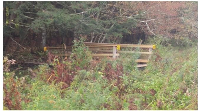
Stockyard trail bridge salvage and reset.
