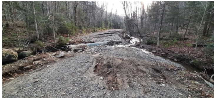
Powley Road Damage Photo Courtesy Craig Small—Piseco Lake, N.Y. USA Facebook
