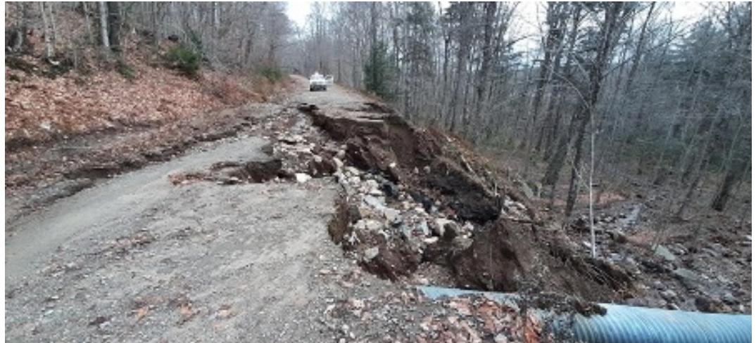
Powley Road Damage
