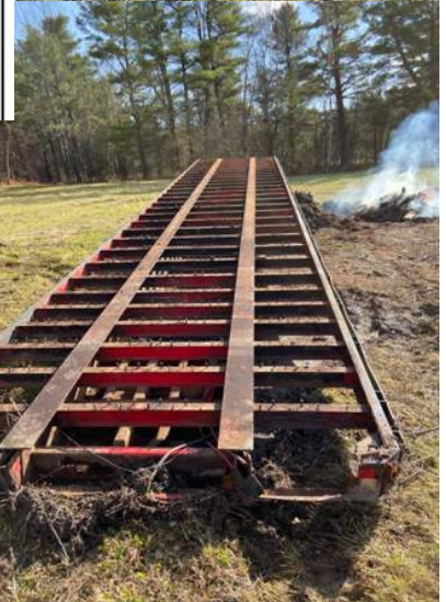
Skip Murrell did the metal cutting and Brian Buchardt removed the old decking. The trailer frame is nearly ready for trail placement. Photo by Brian B.
