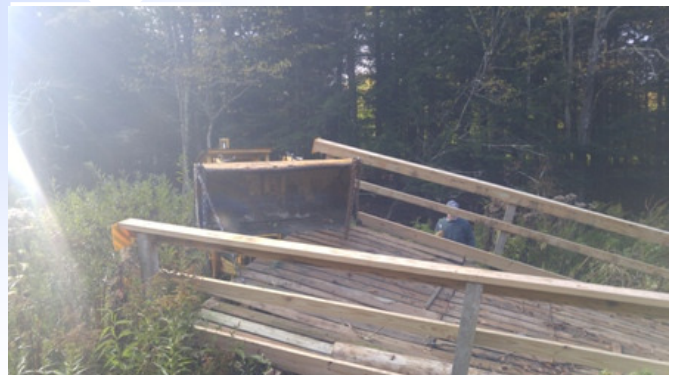
Moving bridge back upstream.
