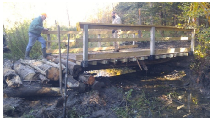
Bridge back in place!
