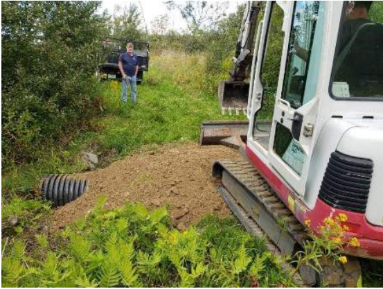
S72 culvert work. Karl Pritchard, Gerry Lenseth, and Brain Buchardt.
