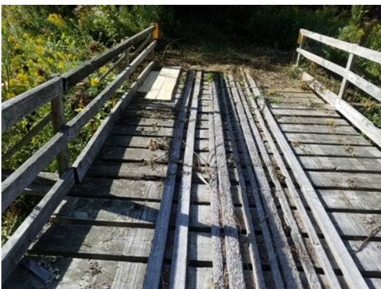
Route 146 bridge on C7B had some decking repaired and guard rails reset. Skip Murrell got the job done. Photo by Skip M.
