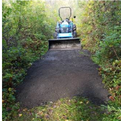
Trail work on S72 to Thacher Park. Photo by Brian B.
