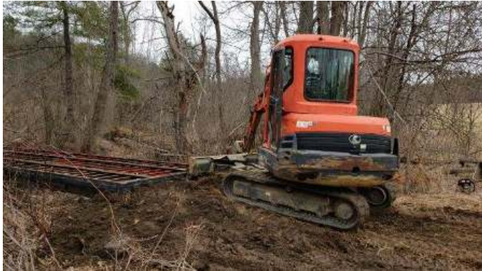
Smoothing the approach ramp.
