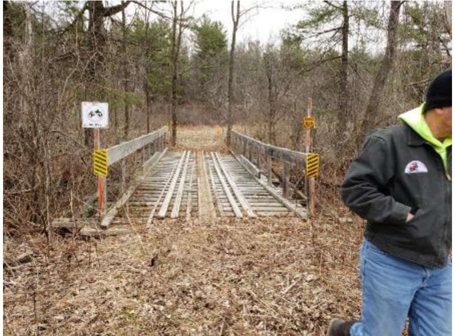
Trail Boss Brian Buchardt makes final inspection before demolition.
