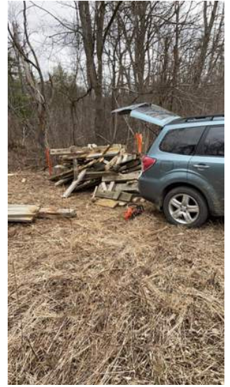
Loading the old decking.
