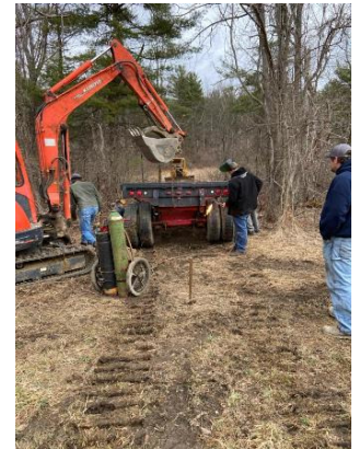
Now the cutting begins.
