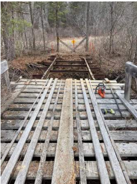
Working across the bridge removing the decking.
