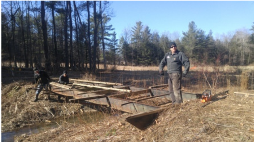
Removing the beam stringers requires good form.
