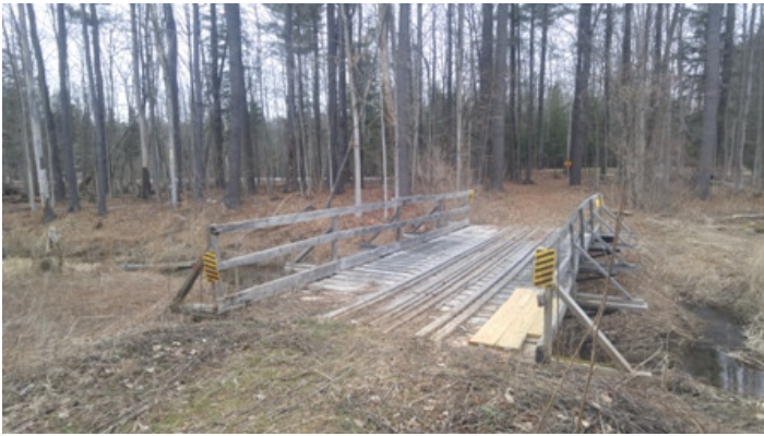
Old decking from original 2010 installation.
