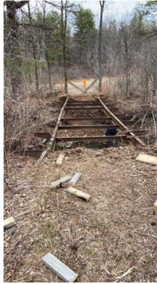
The bare frame exposed.
