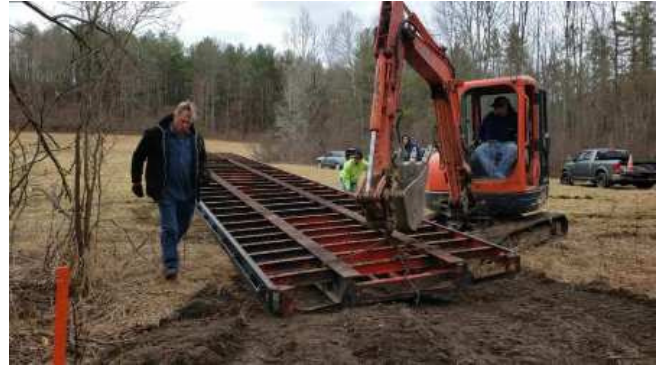
Moving the frame forward.
