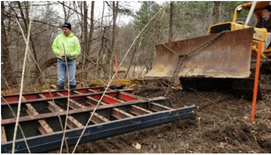
Lifting the far end up onto the abutment.
