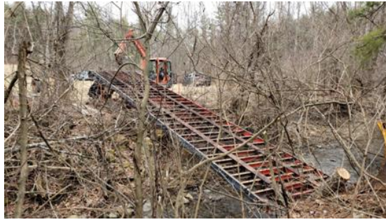
Across but not yet in place.
