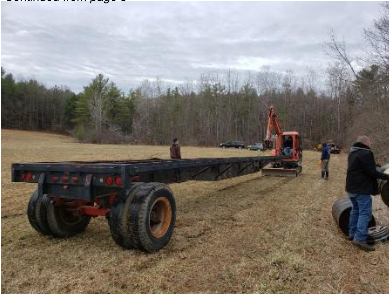
Swinging the trailer frame to the site.
