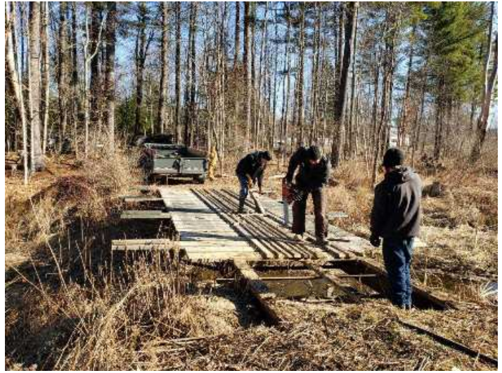
Cutting and ripping up the old decking.
