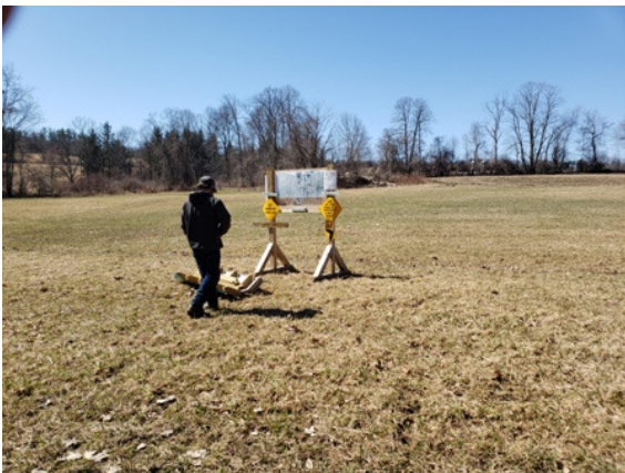
Skip Murrell reports repairing the roof on the C7B/C7G trail junction kiosk in Knox.
