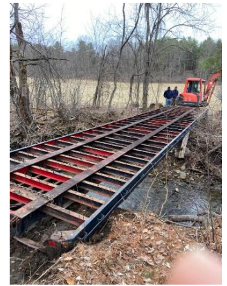
The span across the creek.
