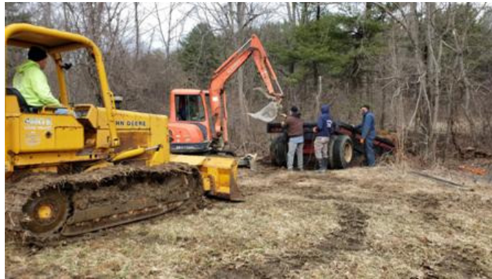
Hoisting the rear axle section for removal.
