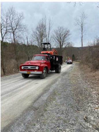
Heavy equipment arrives.
