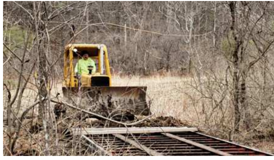
Working the grade on the ramp.
