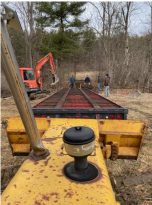
Pushing across the creek.
