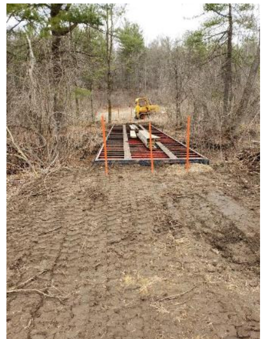
Ready for new decking.
