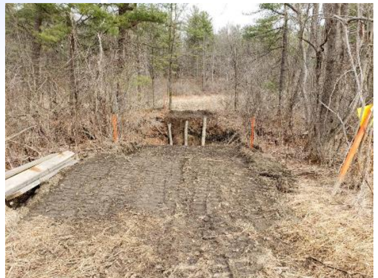
The bridge embankments are readied.
