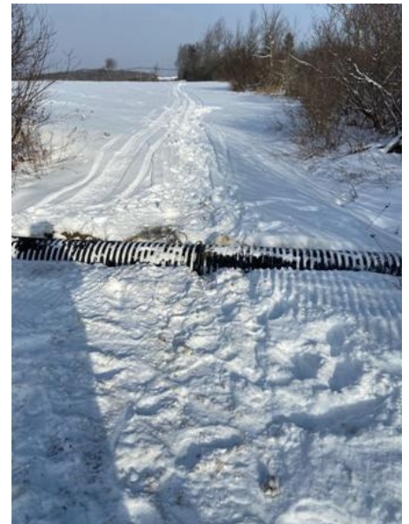
Culvert tube replaced on S72.
