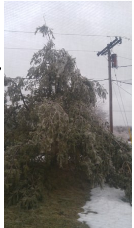
Ice damaged tree hangs low.
