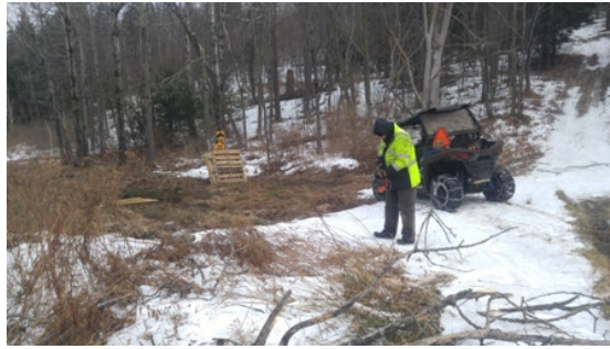
Trail Boss Brian Buchardt clears ice storm damage from trail S72 near Thacher Park.
