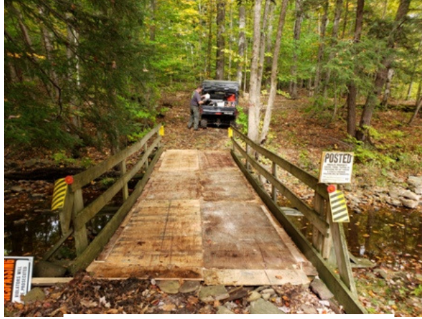
After the temporary decking was installed. The bridge is due for replacement next year. Trail Boss Mark VanWoeart and Skip Murrell got the job done.
