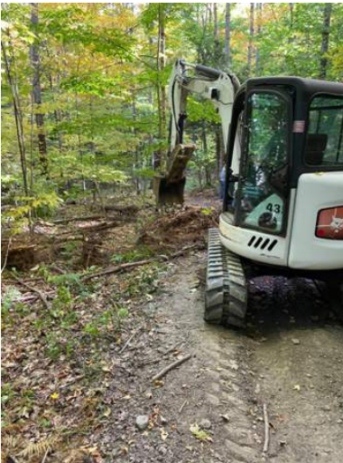
Trail Boss Don Bauer uses a track hoe to clear and widen S73, Maple Inn trail. Helping out were Keith Kodra and Alex Gibitz.
