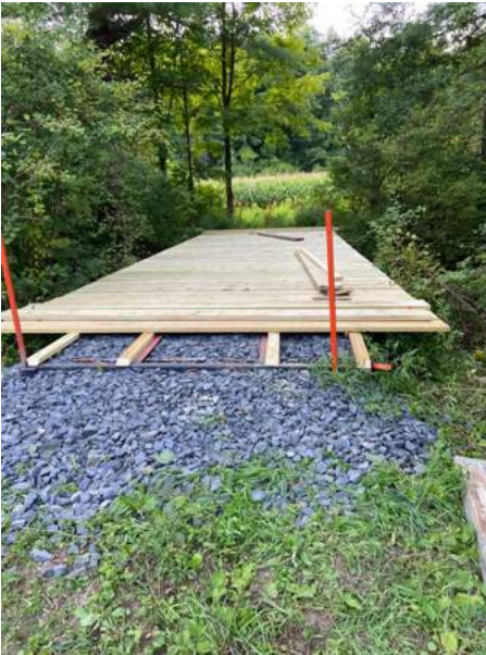
Decking is finished, awaiting runners and railings. Finished bridge, weight testing.
