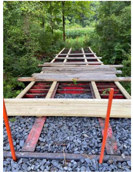
Nailers are attached and decking starts
