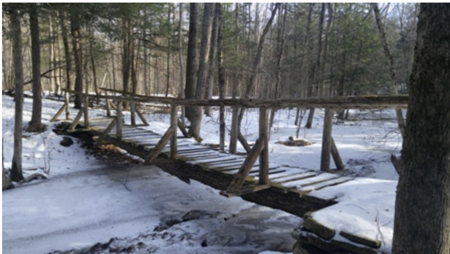
The old foot bridge at the end of it's useful life. A new bridge able to support snowmobiles and grooming equipment was needed to provide safe crossing of the stream in the Charleston State Forest.
