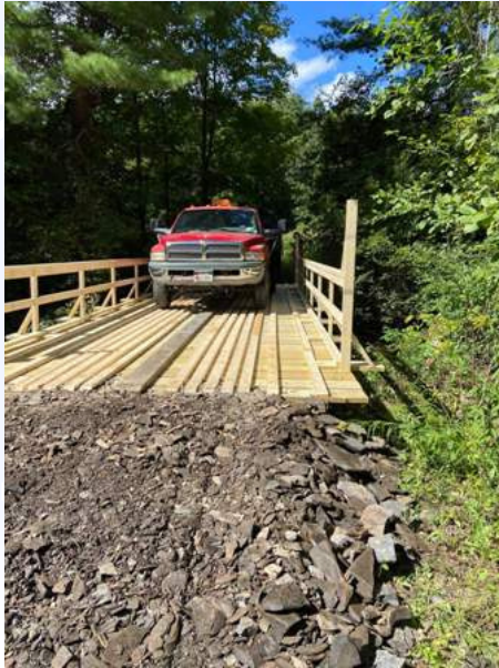
Decking is finished, awaiting runners and railings. Finished bridge, weight testing.
