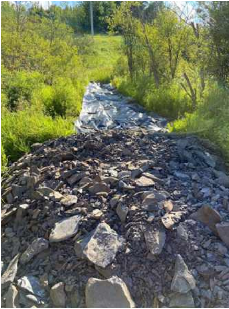
Spreading 9 loads of shale over reset culvert will greatly improve riding conditions.
