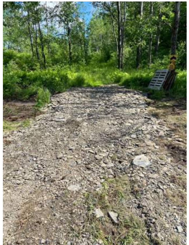
Shale and a culvert will help keep snowmobiles up and out of the spring fed water areas on S-72 enroute to Thatcher Park.
