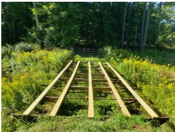
Decking nailers have been put on the Rt 146 bridge. Bridge is to be decked in the near future. Photos by Skip Murrell.
