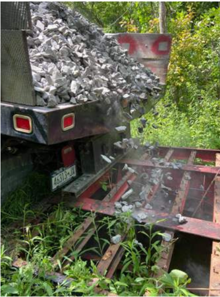
Dropping shale to secure the footing.
