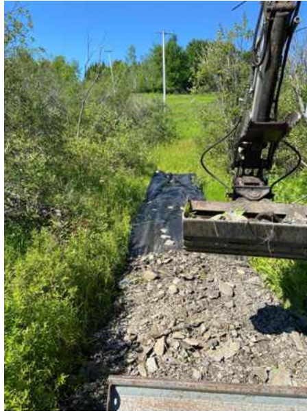
Spreading 9 loads of shale over reset culvert will greatly improve riding conditions.
