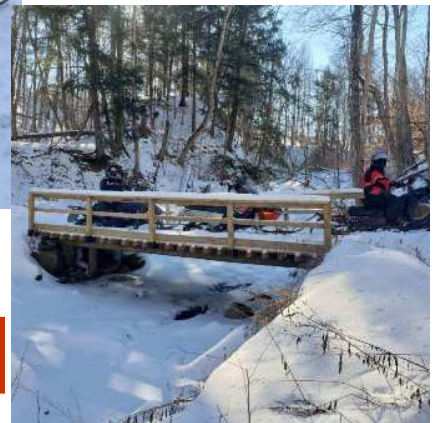
Crossing the Irish Creek bridge on C7E.
