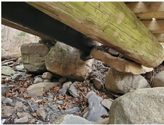
The footings for the bridge over Irish Creek needed reinforcement. Before and after pics by Trail Boss Tom Rulison.
