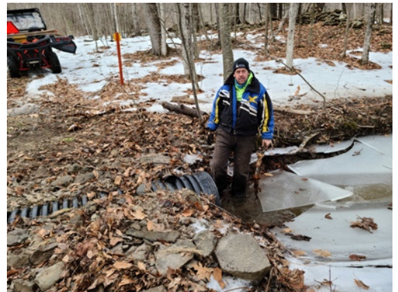
Trail Boss Brian Buchardt clears a clogged culvert on C7B near Ostrander Rd.
