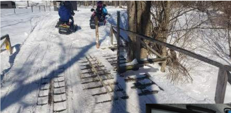
Club members stop to mark a broken deck board on the Knox Ball Field bridge.
