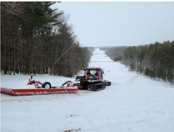
C7B - gas line above Rt 146
