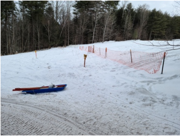
Snow fencing had to be added across pipeline in Wright.
