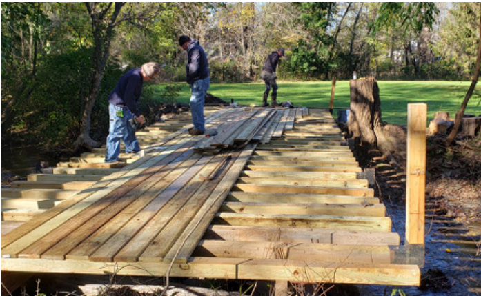
It was an all day job getting the deck, wear boards and railings up.
