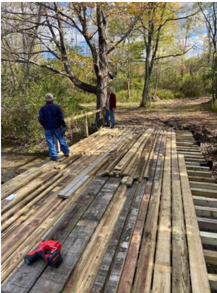
It was an all day job getting the deck, wear boards and railings up.
