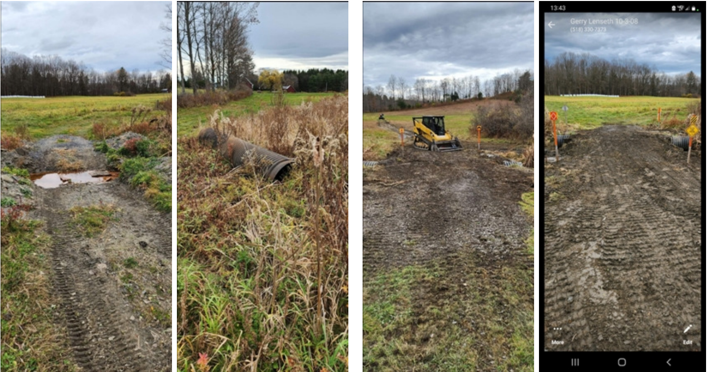
Resetting a culvert on C7B near Weaver Rd. Photos by Eric Dubb.
