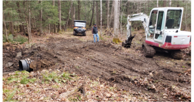
Karl Pritchard reinstalled the culvert behind the Demis property in Knox
