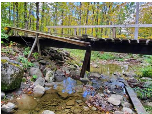
The Esperance Ball field bridge on C7E suffered damage when it's hand railing was smashed off on one side. Photos by Trail Boss Tom Rulison.
