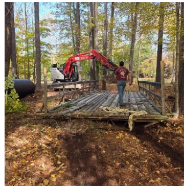
Stripping away the rails and decking.
