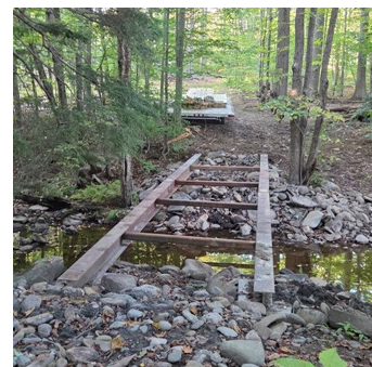
Bridge frame ready for decking.
